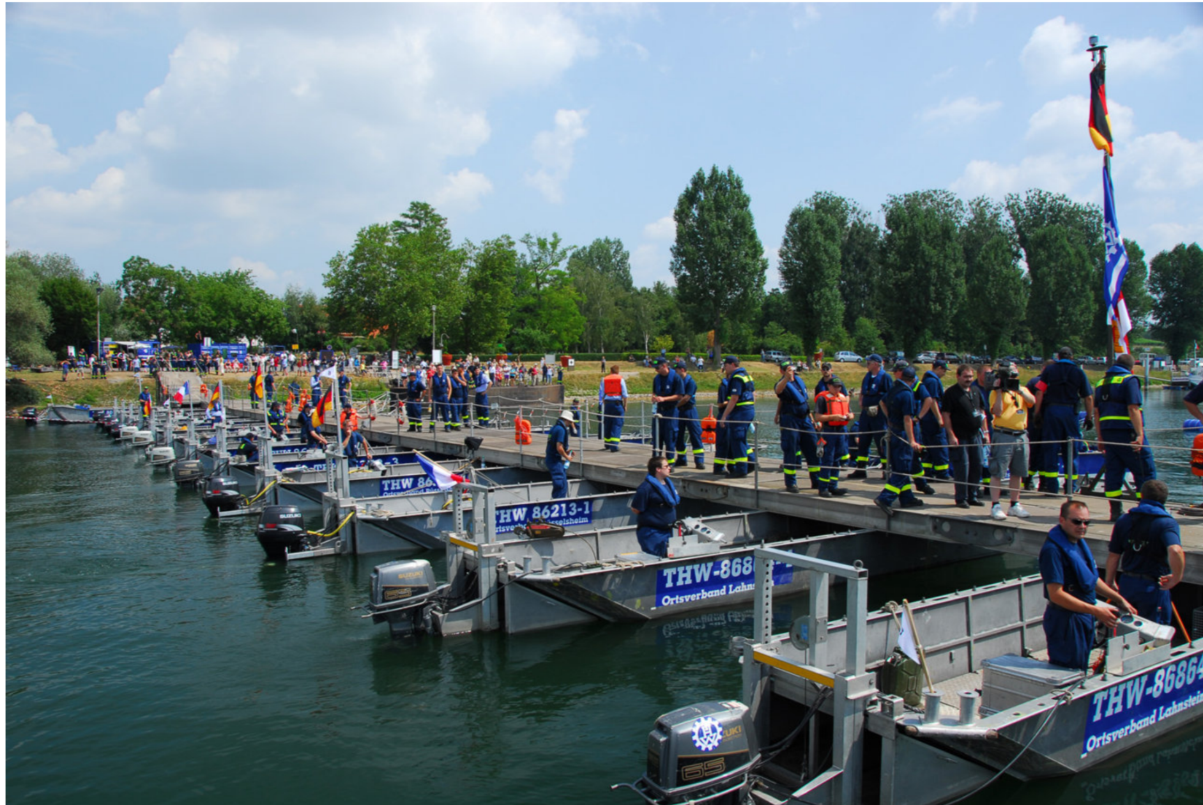
Juli 06: construction of a 200 meter pontoon bridge in Breisach over river Rhine
