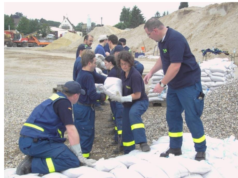
Training for construction of a bank with sandbags
