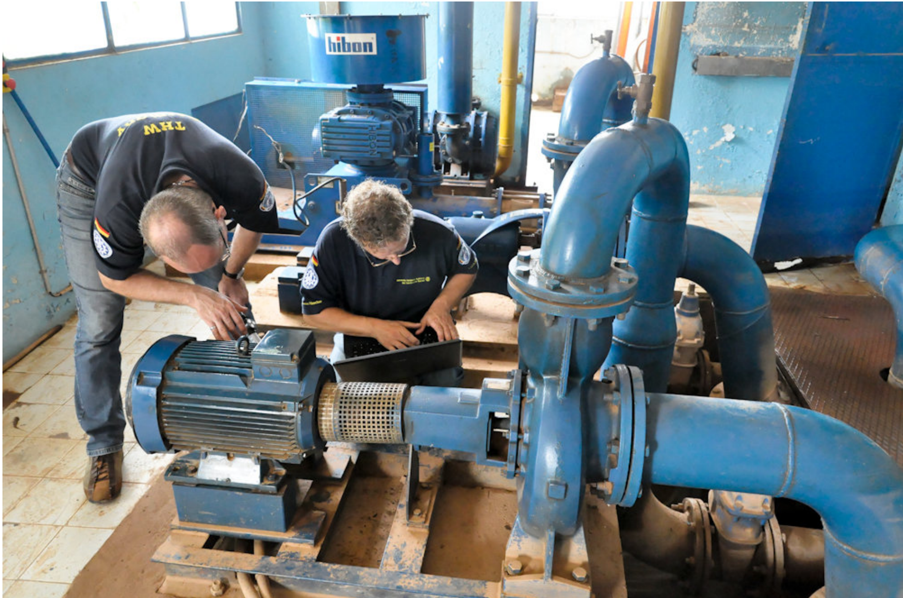
An electrical plant was destroyed, a water plant was flooded
