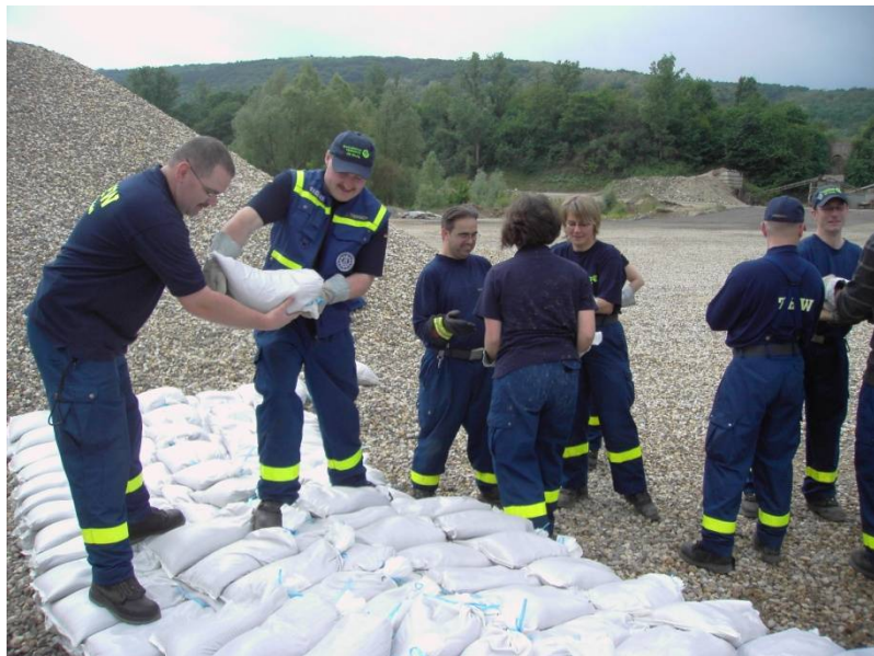
Training for construction of a bank with sandbags
