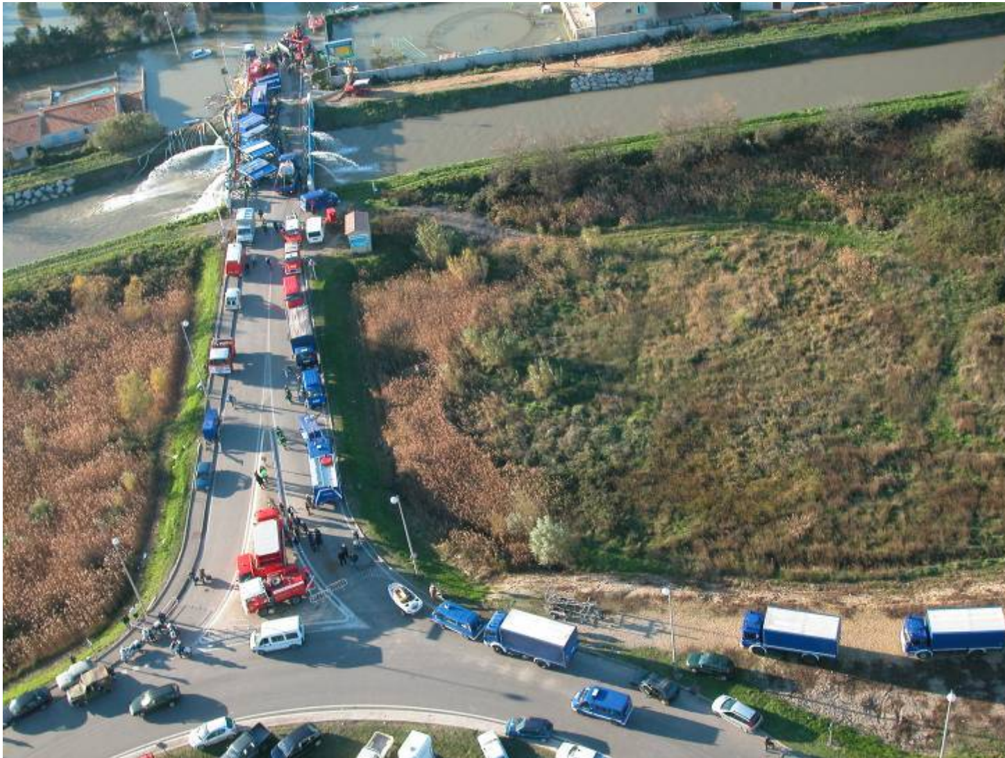
Flooding in December 2003.
