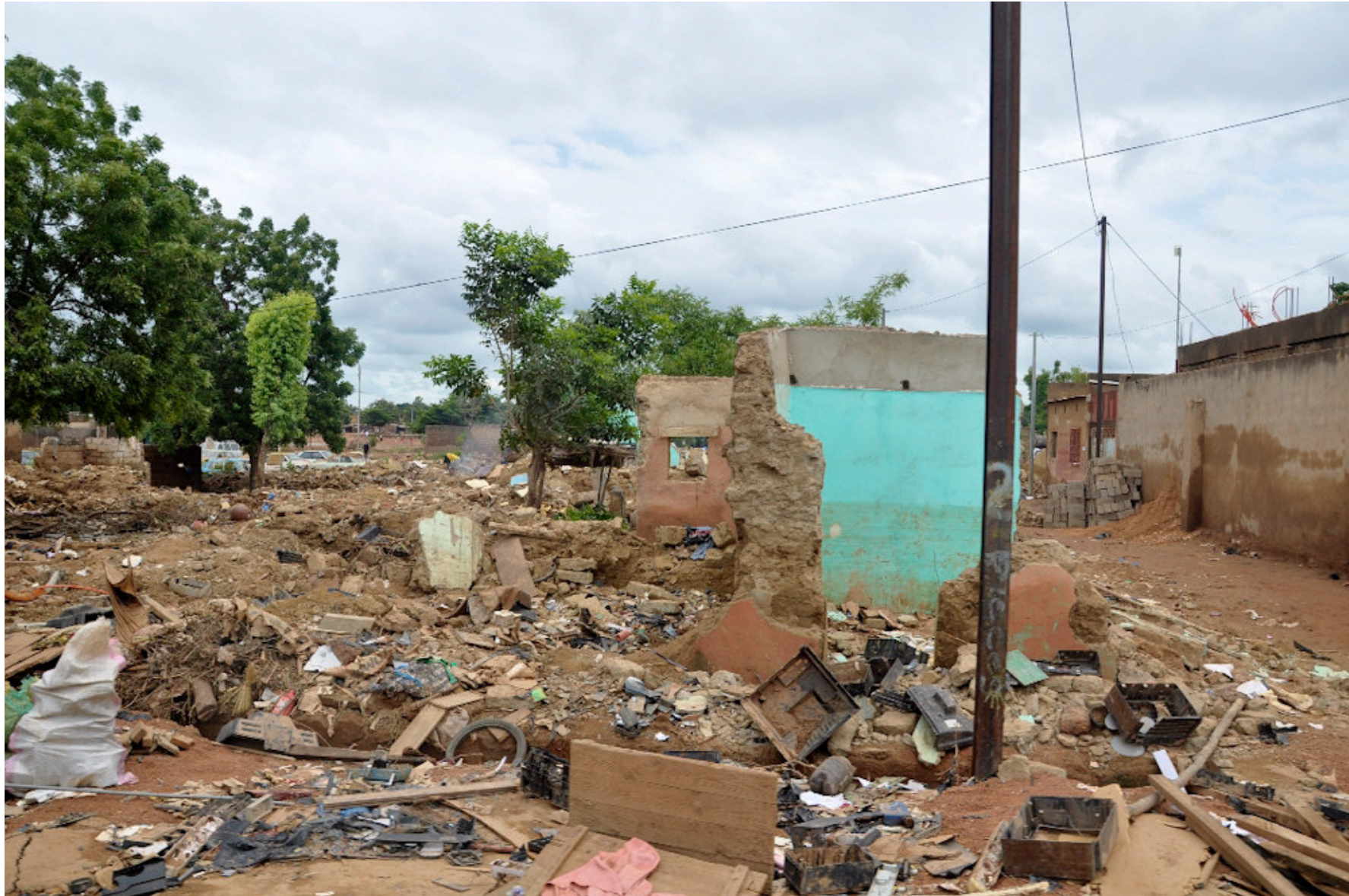
5 victims, Roads, bridges and dams have been badly damaged
