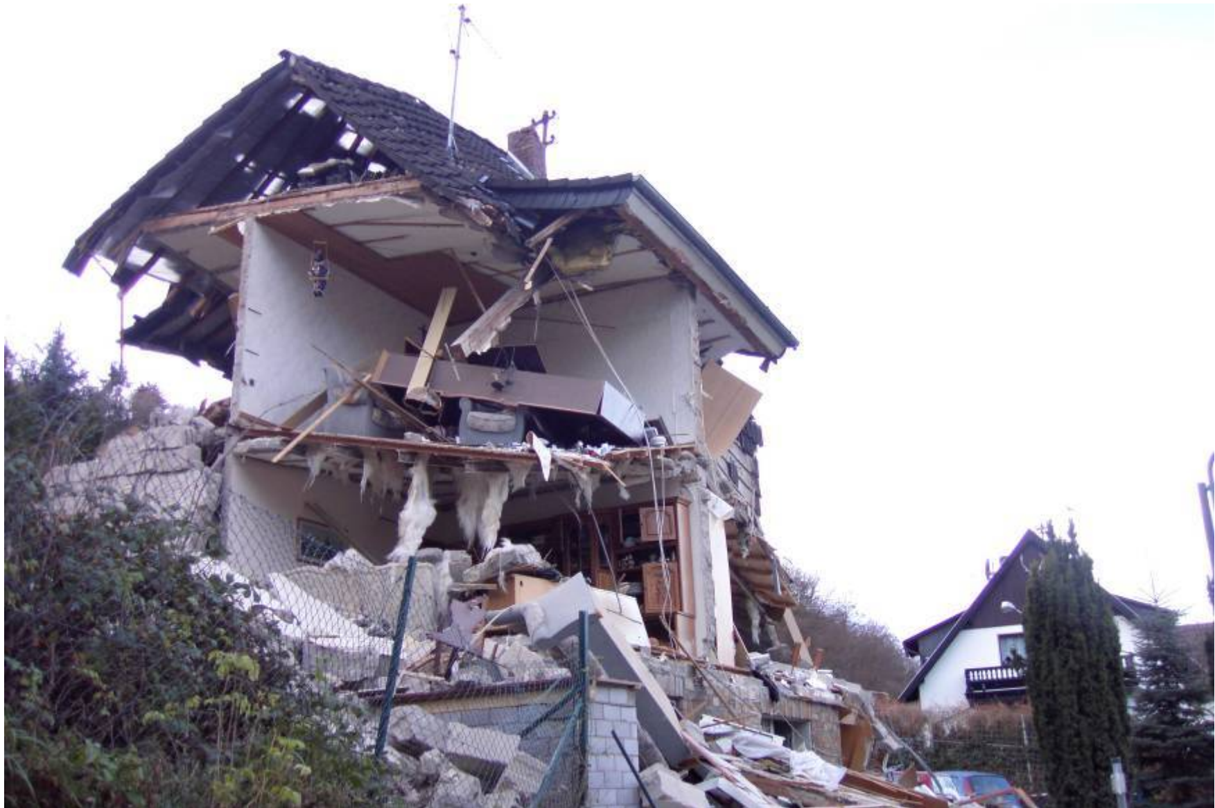
December 2003, Gas explosion in Oberzissen
