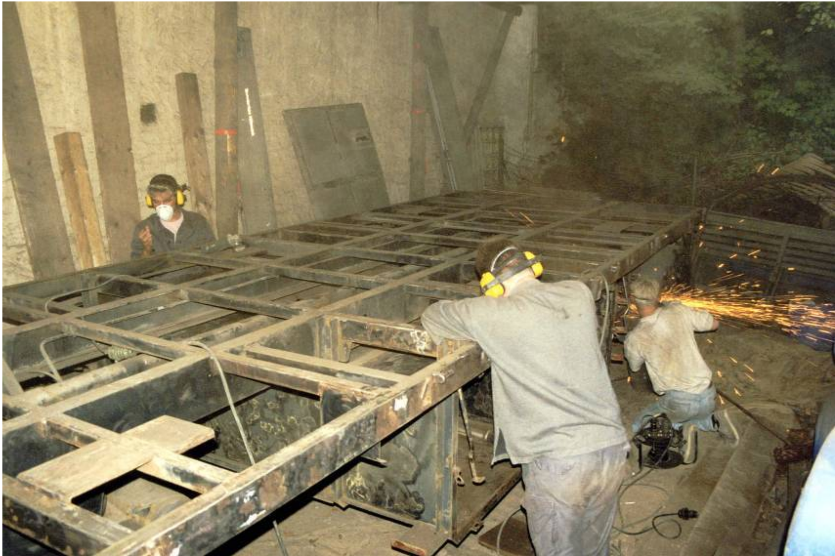
Grinding, priming and painting of a trailer
