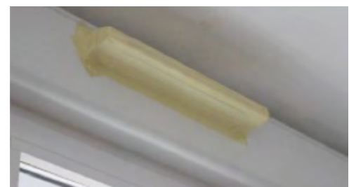
Sealing of an aerator on a window in the living-room
