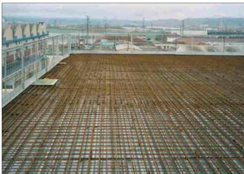
Losa in situ
