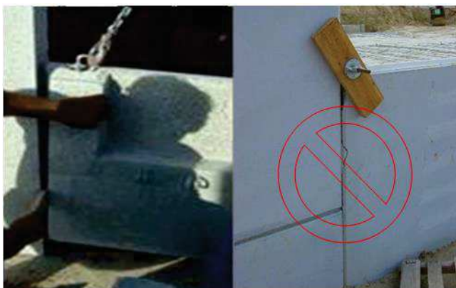
BADLY EXECUTED VERTICAL JOINTS
