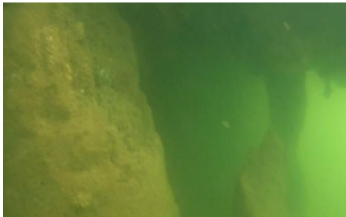
Figura 31. Pila 1. Cavity under the pile of pile 1
