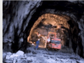
TEAM SL Tunnel P
