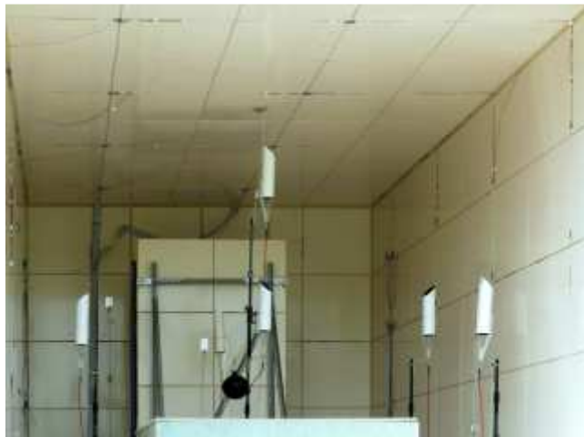
Fig. 2 Installation of HFS Tiles.
