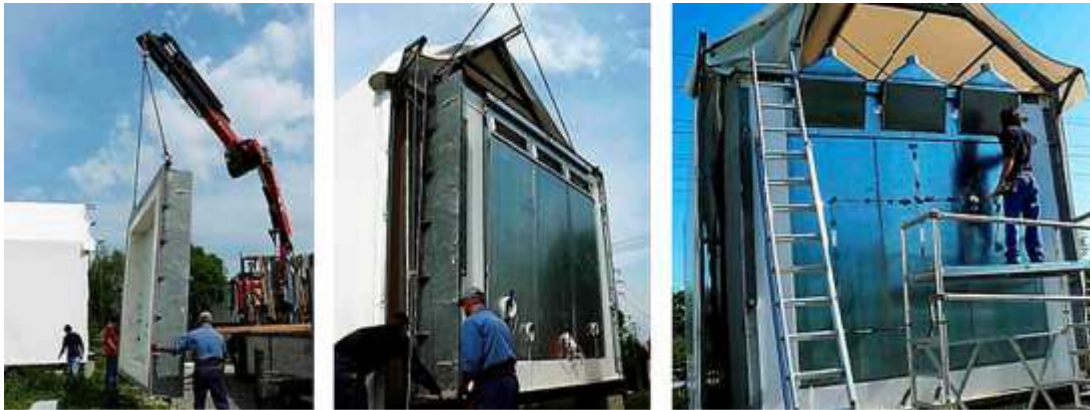
Figure 9 - Movement and installation of the sample in the test cell
